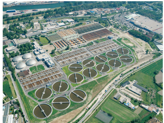
Figure 1, wastewater treatment plant. This treatment plant receives wastewater from a network of lift stations, each of which must be controlled and monitored to assure correct operation.
