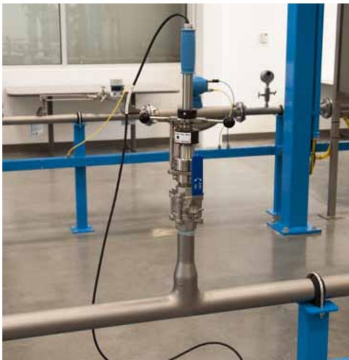
*Figure 5: An example of a pH sensor installation in a convenient location for maintenance by plant personnel.*
