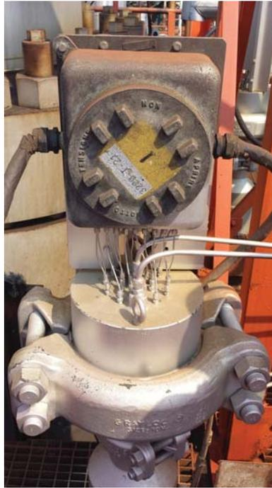
*Figure 3: An enclosure contains either a terminal block that sends sensor data via the thermocouple cable to the control system or a transmitter that sends sensor data via 4-20 mA signals to the control system.*
