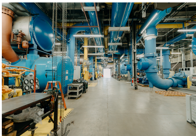
Citizens Energy Group's process consists of numerous 5,000-ton chiller systems (left)
