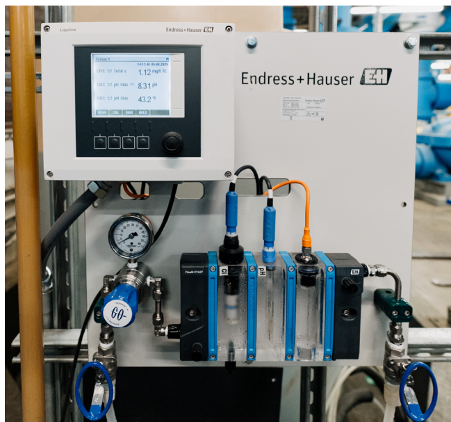
Endress+Hauser and George E. Booth Co. worked with Citizens Energy Group to provide a total chlorine panel, comprised of the digital total chlorine sensor Memosens CCS53E, digital pH sensor Memosens CPS11E, Liquiline CM44X transmitter and the Flowfit CYA27 assembly
