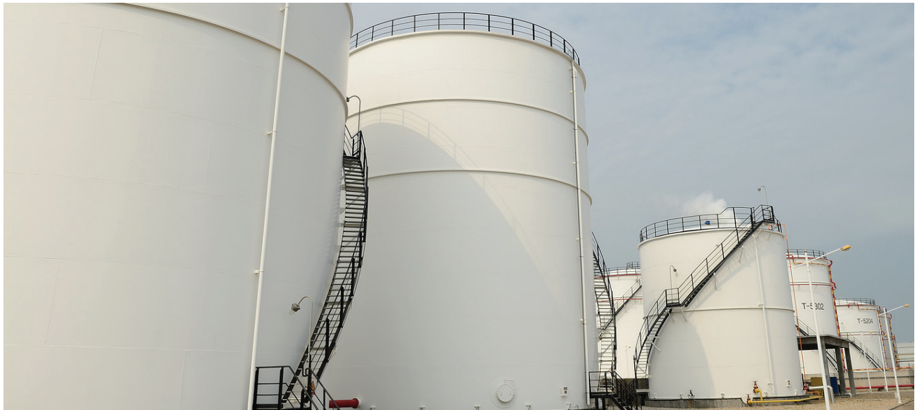
Figure 1: Storage tanks containing dangerous chemicals require multiple levels of instrumentation, controllers and software that can monitor the contents of a vessel and provide an alarm in the event of a leak or overflow event.
