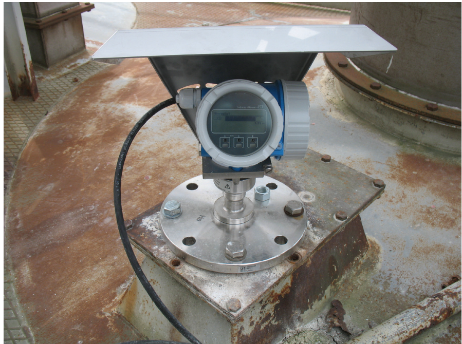
FIGURE 3. The Endress+Hauser FMR57 26GHz level instrument has an air purge connection, multi-echo tracking and a small 4-inch antenna to accurately measure level in a silo up to 230 feet tall.
