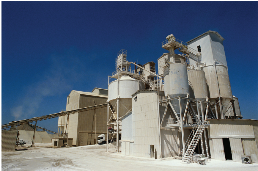
FIGURE 1. Circular clinker silos used to store cement, concrete and similar materials pose problems for traditional level measurement instruments.
