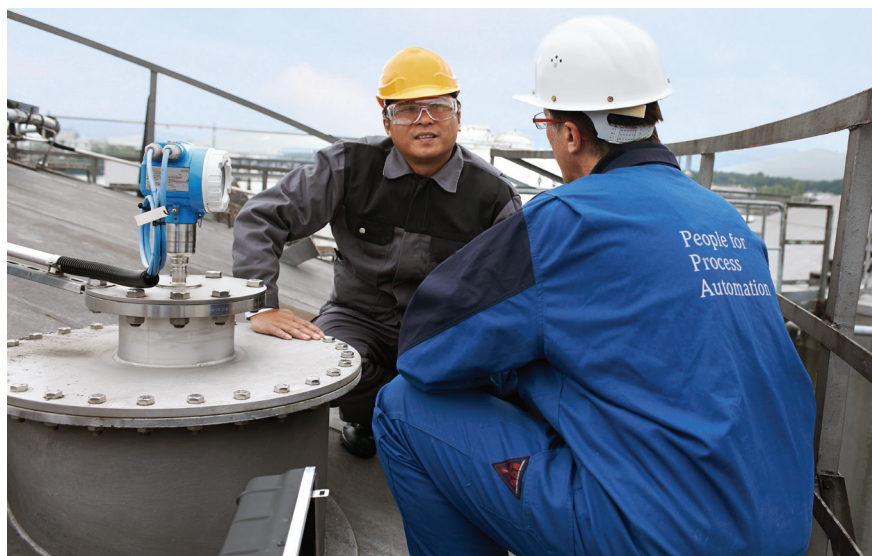
FIGURE 1. Radar level instruments have the necessary accuracy for custody transfer applications.
