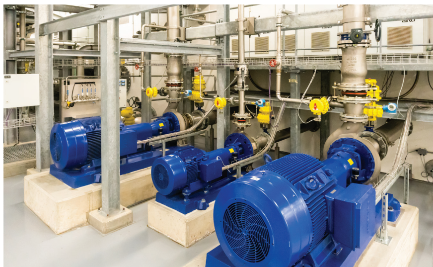
FIGURE 1. With smart pumping, cascading pumps from large reservoirs ensure required flow rates are achieved reliably and efficiently based on system demand.
