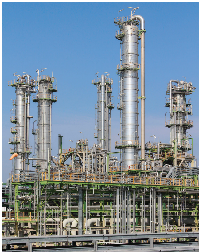
Figure 1: A catalytic reforming unit converts naphtha into high-octane aromatic compounds.
