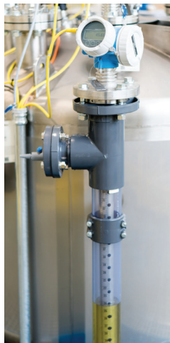
Figure 5: Endress+Hauser Levelflex FMP55 transmitters were installed on this separator in the oil inlet and outlet streams
