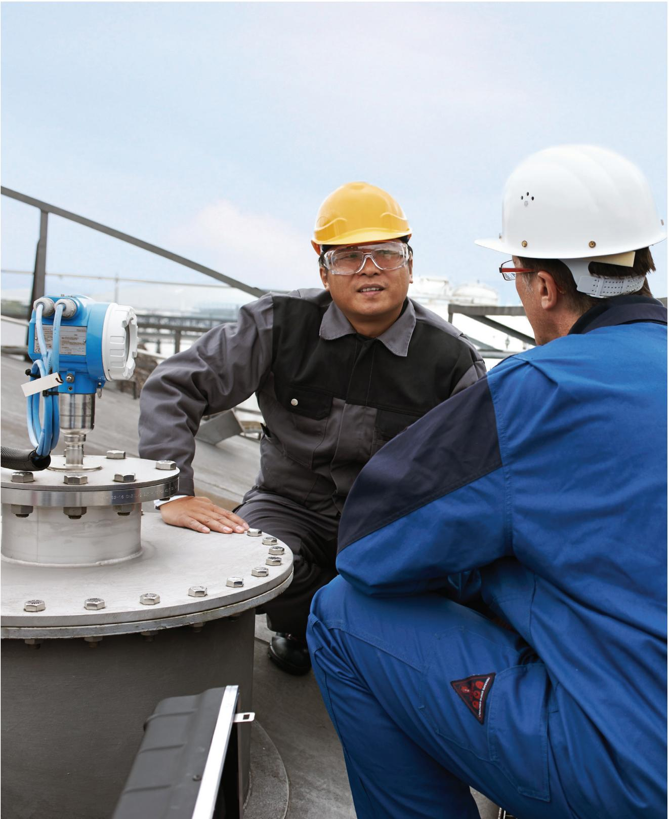
*Figure 6: Ideally, a radar instrument should be installed as close to the silo wall as possible, given the limitations imposed by the beam angle and the size of the hole needed to mount it*
