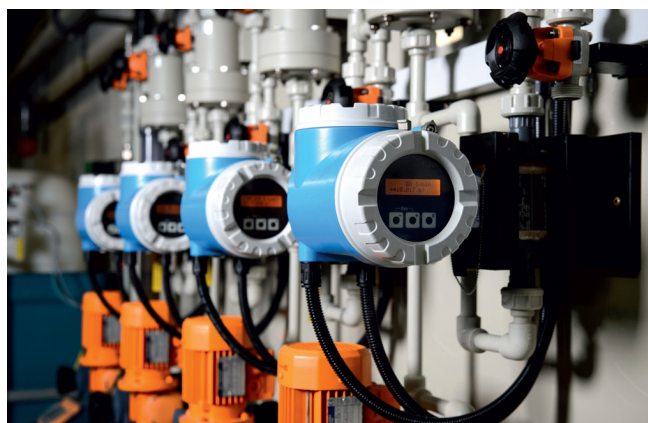
Figure 1: Modern instrumentation provides diagnostic and status information and specialty software helps the maintenance department use it for preventive maintenance.
