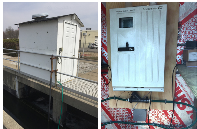
Figure 3: Heated/ventilated analyzer shelter with 3/4" hose in from submersible pump with bypass back to process. Y strainer, under analyzer, with 3/4" hose inlet/outlet and analyzer connection. Optional integrated reagent cooling module extends reagent life to maximum while also eliminating the need for air conditioning for ambient temperatures up to 104°F (40°C).
