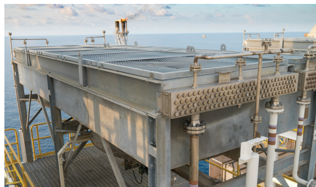
Figure 2: Fin fan heat exchanger coolers are used to cool distillates.
