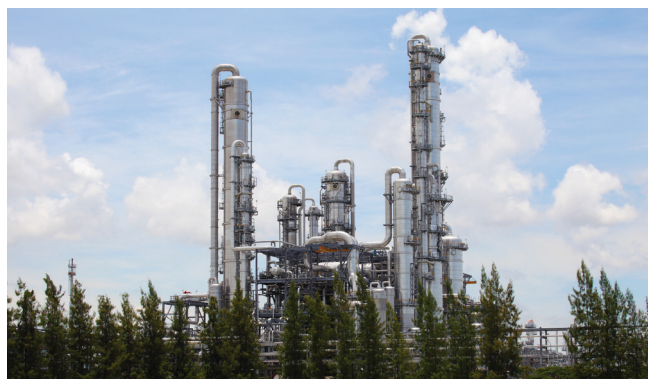
Figure 1: Thermocouples and RTDs are used in distillation column cooling processes.
