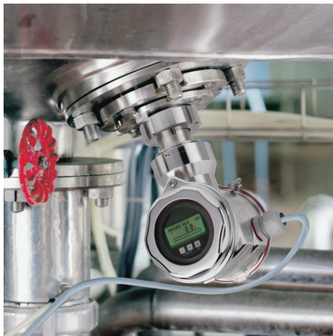
Figure 1: Pressure instruments in the food and beverage industry are subject to drift from condensation and temperature.
