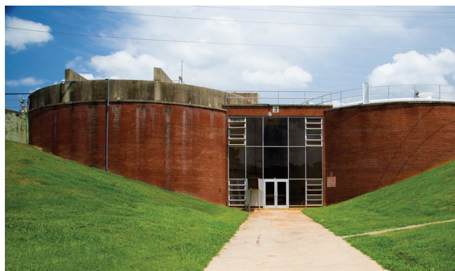
Figure 1: Anaerobic digesters in Charlotte, NC, treat sludge and generate biogas, which can be used to generate electricity.
