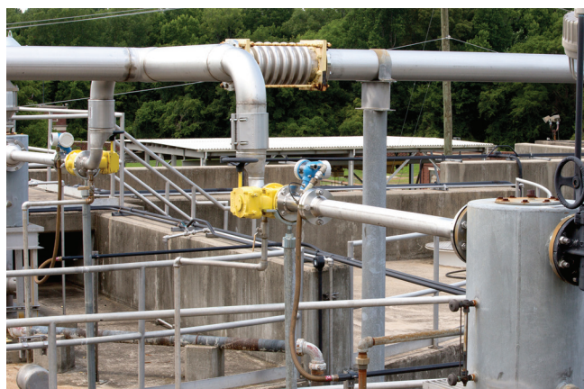
Figure 3: The City of Charlotte installed Proline Prosonic Flow B 200 ultrasonic flowmeters from Endress+Hauser in 2013.
