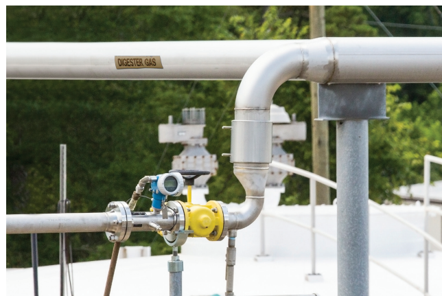
Figure 4: Typical installation at the City of Charlotte. The B 200 has an integral temperature sensor to help compute the methane fraction of the biogas.
