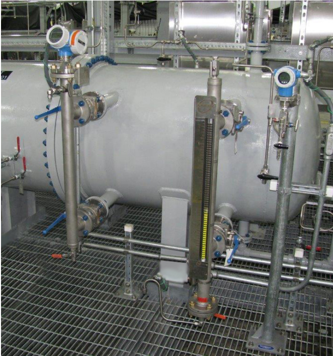
Figure 2: Horizontal oil-gas-water separator.
