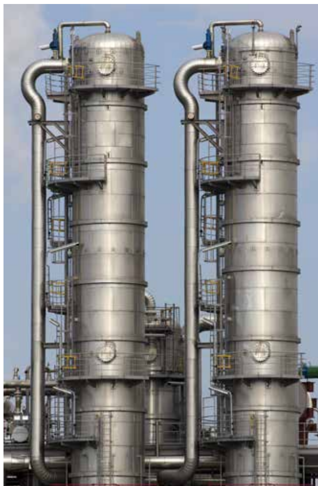
Figure 1: A catalytic reforming unit converts naphtha into high-octane aromatic compounds.
