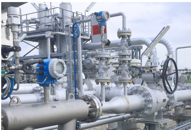
Figure 1: Flowmeters like those shown here can play key roles in reducing risk with safety instrumented systems (SIS).
