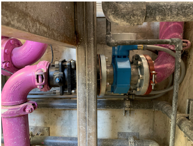
The Promag W 400 is easily installed directly in-line to provide accurate data with no pressure loss
