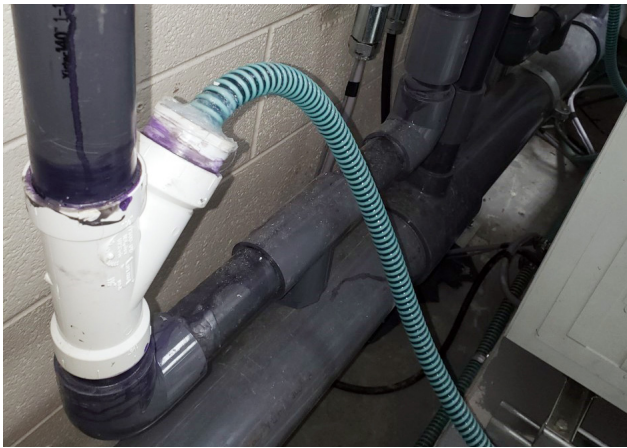
Flow through attachment for pulling sample process out of the line and into Endress+Hauser sampler.
