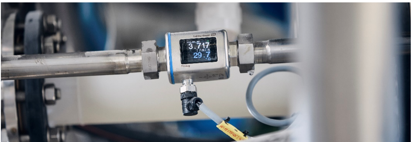
Figure 1: An Endress+Hauser Picomag electromagnetic flowmeter digitally transmits primary and secondary process variables—plus instrument diagnostic data—to a central host system via IO-Link.
