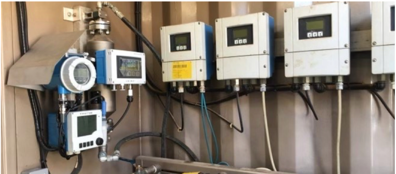
Figure 3: The Proline Promass I 300 Coriolis flowmeter by Endress+Hauser transmits multiple process values and instrument diagnostic data via HART, WirelessHART and Bluetooth.
