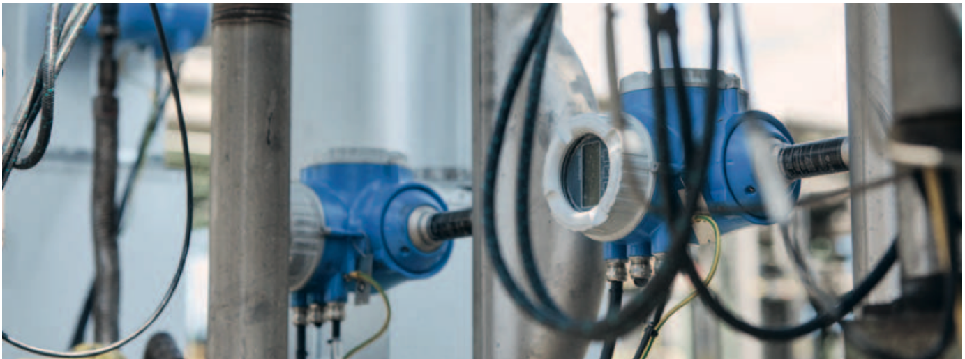
Figure 1: Endress+Hauser Promass F 300 mass flowmeters with Heartbeat Technology provide self-diagnostics and support in situ testing and verification.
